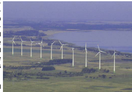
The Osorio windfarm (above) is located in Osório, Rio Grande do Sul. It comprises 75 wind turbines with an installed capacity totaling 150MW. Commissioned in 2006, it can supply a city of 700,000 people.
