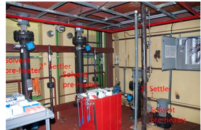
Deasphalting pilot under construction
