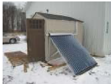
Evacuated tube solar collector
