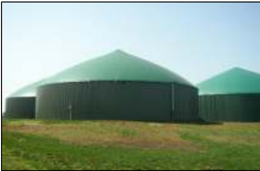
Completely Stirred Tank Reactor (CSTR)
